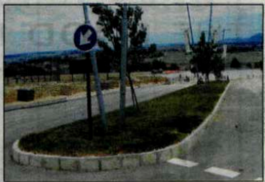
The revamped road network at Lanseria International Airport. Photo submitted.
