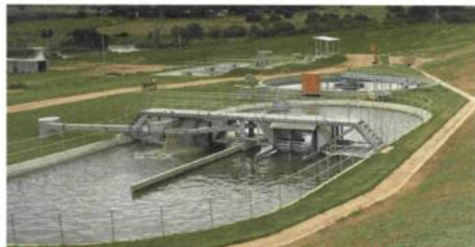
Expert wastewater treatment works (WWTW) at Lanseria Corporate Estate. Photography courtesy of Tecroveer
