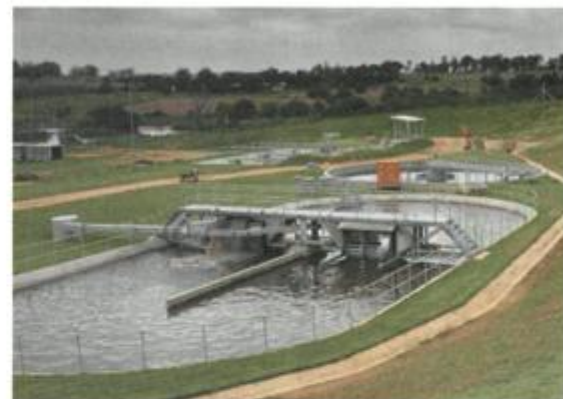
Secondary settling tank situated between pasveer reactor in the foreground and head of works behind it
