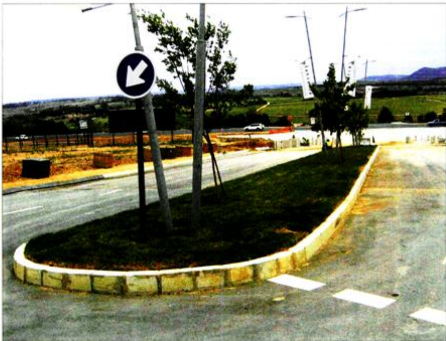
Road upgrades surrounding Lanseria Corporate Estate
